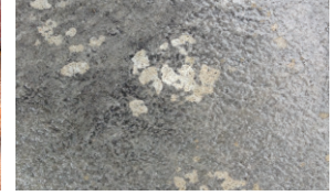
Accumulating moisture under excess sealer can cause a weak layer of concrete paste to disbond.
