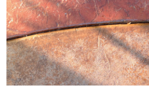
"Whitening" or "frosting" is a sign that sealer has delaminated due to excess moisture and/or excess sealer.
